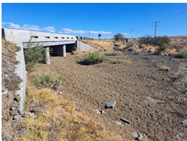
Road crossing with culvert
