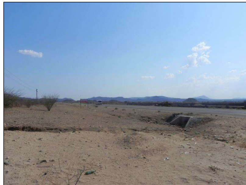
Figure 7-90: View along the D4190.
