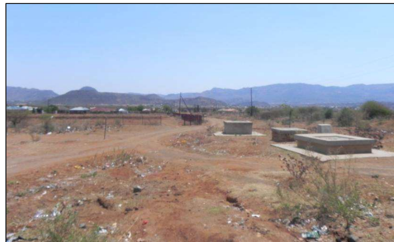
Figure 7-82: Scour boxes next to the R37, at the eastern section of the alignment.
