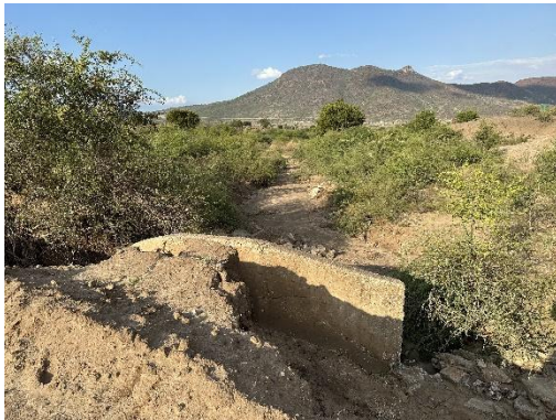
Figure F2: Drainage line in the focus area close to access point 1-10
