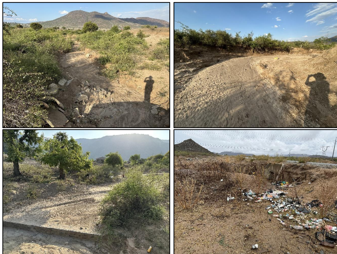
Photograph notes: Top left: View of the channel and riparian zone of the drainage line downstream of the existing road close to the access point 1-10; Top right: The channel of the drainage line near access point 1-13 displaying accelerated bank erosion; Bottom left: Residual riparian trees that have been felled along the drainage line upstream of access point 1-13; Bottom right: Dumping of refuse in the riparian zone of the drainage line denuded of vegetation at the access point 1-08.
