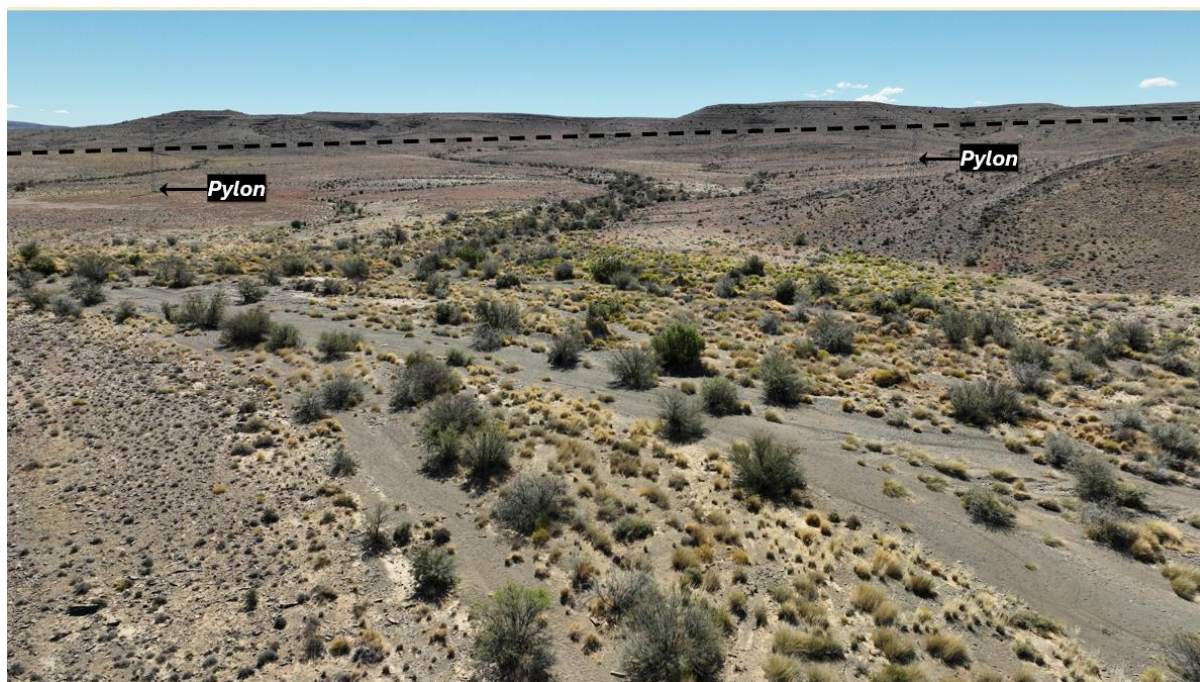
Figure 14. Typical power line route (dashed line) approximately 50 km east of Laingsburg across an unnamed tributary of a medium-sized drainage line. Pylons are indicated outside of watercourses and riparian zones and access is very limited for maintenance with no clear existing tracks (Coordinates: 33° 4'31.23"S, 21°25'42.52"E)
