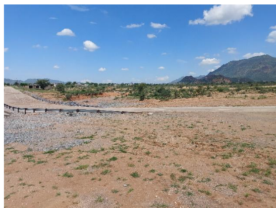
Figure 11: One of the more recent bridges constructed by the Local Community
