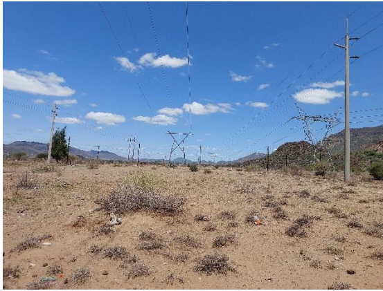
Figure 4: Electrical Infrastructure within the Proposed Pipeline Route
