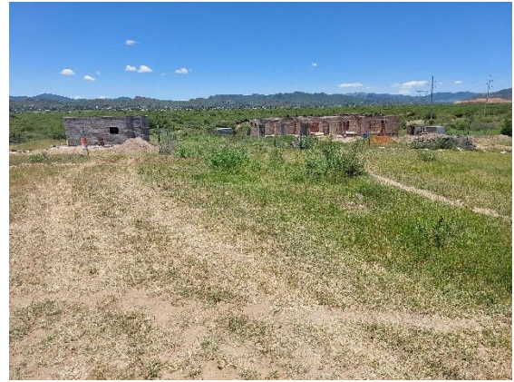
Figure 5: Houses under construction within the Project Area
