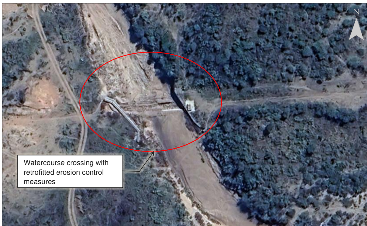
Figure 2-16: Underground pipeline crossing (June 2023), with the erosion control measures
