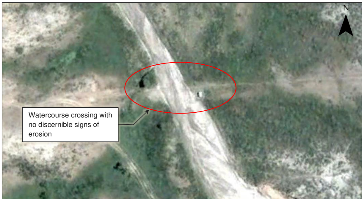
Figure 2-14: Aerial view of a nearby underground pipeline crossing from January 2007
