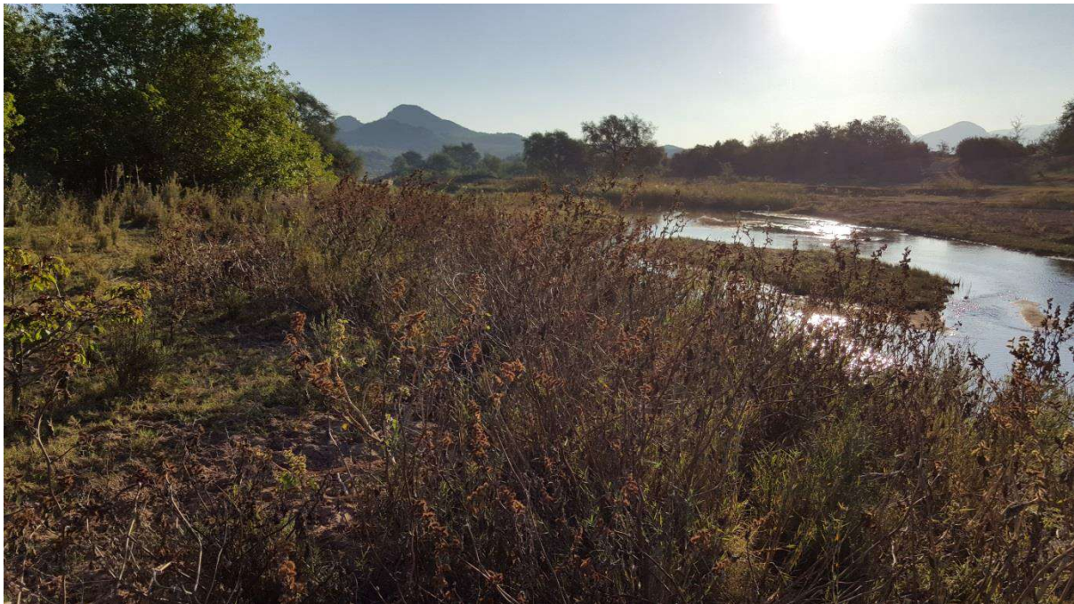
Figure 4-2 View from left bank looking downstream at the pipe crossing site
