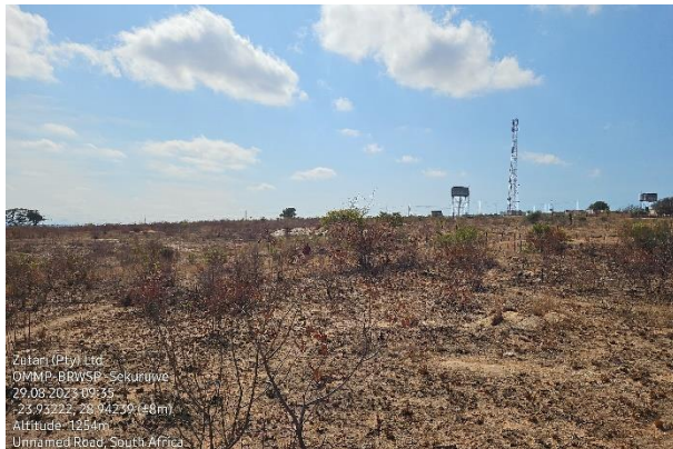
Figure 22: Nearby water tower infrastructure
