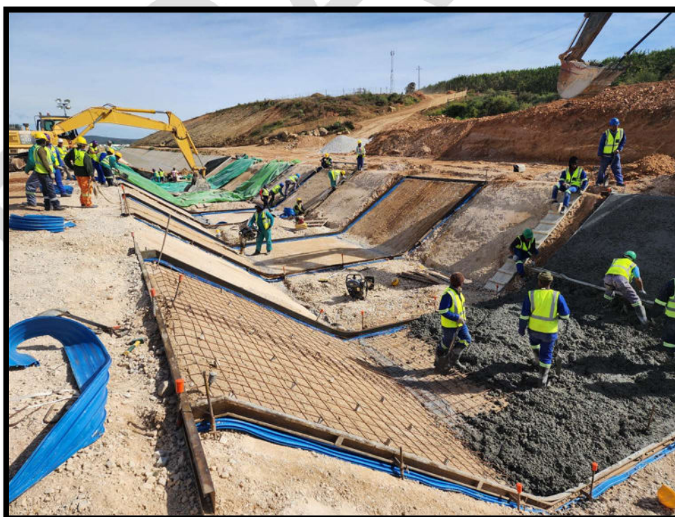
Figure 26. Example of replacement work on a canal (photo: C Jonker)
