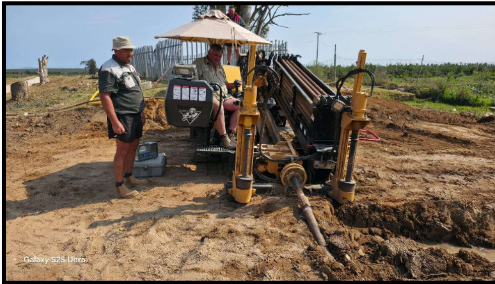
Figure 31. Horizontal Drilling process (photo: C Jonker)
