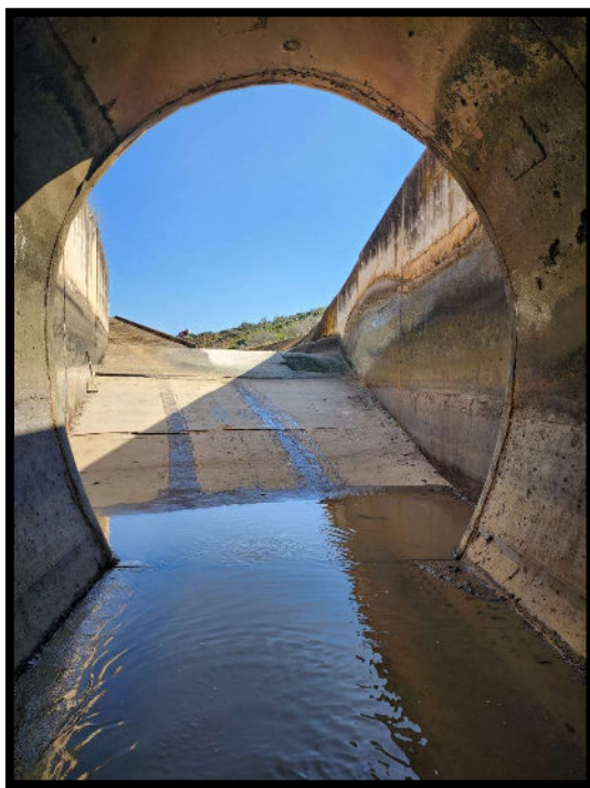
Figure 20. Entrance of the tunnel looking out towards the open canal (photo: C Jonker)
