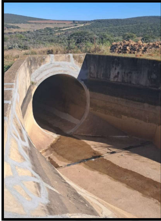
Figure 21. View of the outlet of the Scheepersvlakte syphons (photo: H Forbes)
