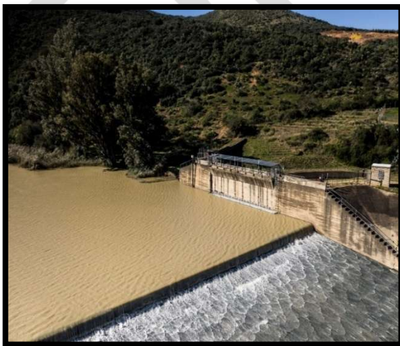
Figure 8. Bird's eye view of Korhaansdrift Weir looking at the sluice gates (source: LSRWUA)
