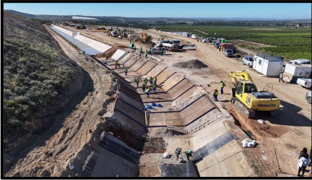
Figure 27. Example of works undertaken to replace canal panel (photo: C Jonker)
