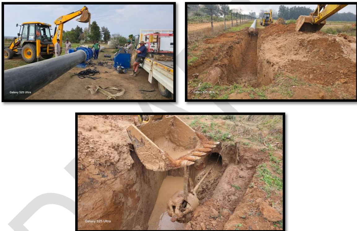
Figure 32. Combination Technique for Solid Wall Polyethylene Pipe (Photos: C Jonker)
