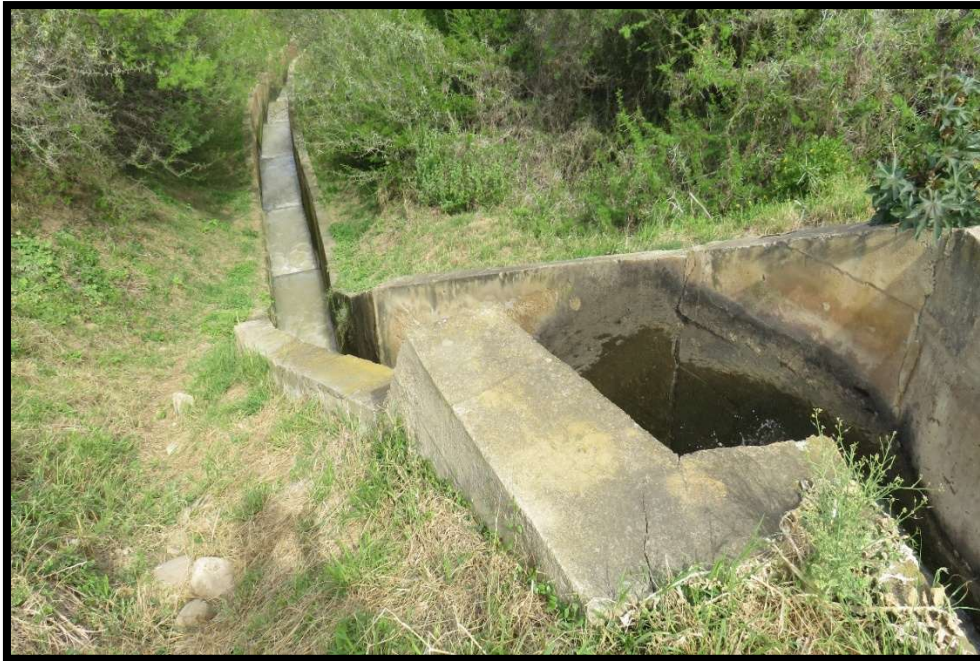
Figure 14. Reject at Barkley Bridge (photo: T Duvenhage)
