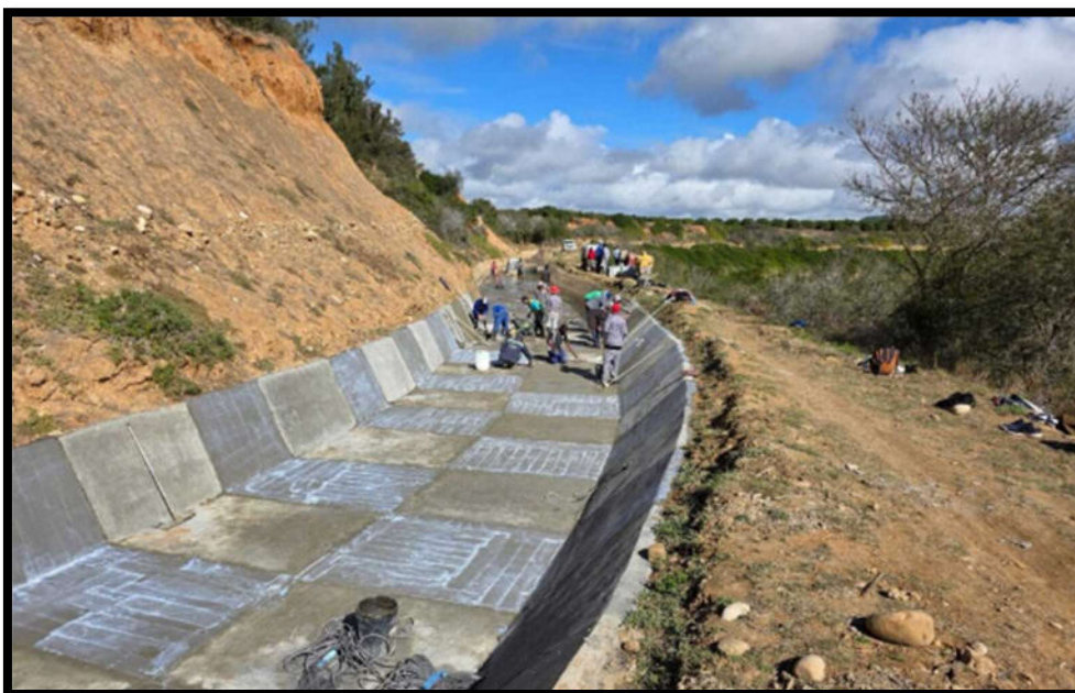
Figure 25. Example of canal sealing (photo: C Jonker)
