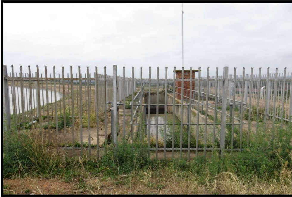
Figure 19. Typical masonry structure associated with telemetry installations (photo: T Govender)
