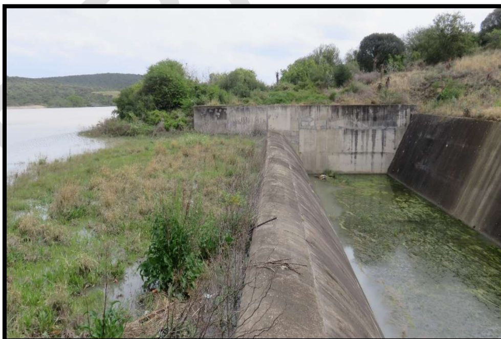
Figure 12. Spillway at Scheepersvlakte Dam (photo: T Duvenhage)
