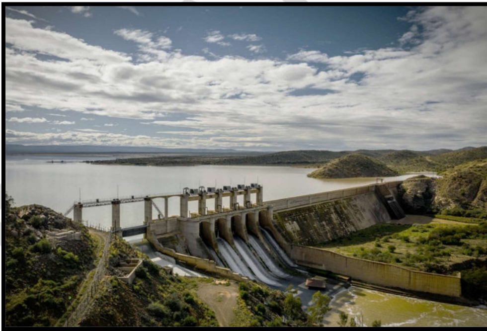
Figure 5. Bird's eye view of Darlington Dam (source: LSRWUA)
