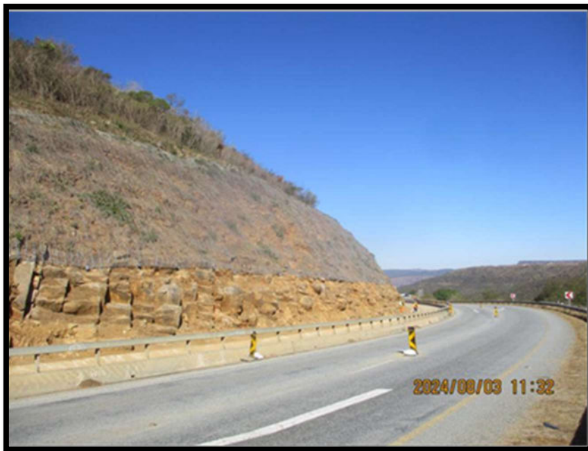
Figure 35. Example of ground anchors and mesh (Source: A Nel)
