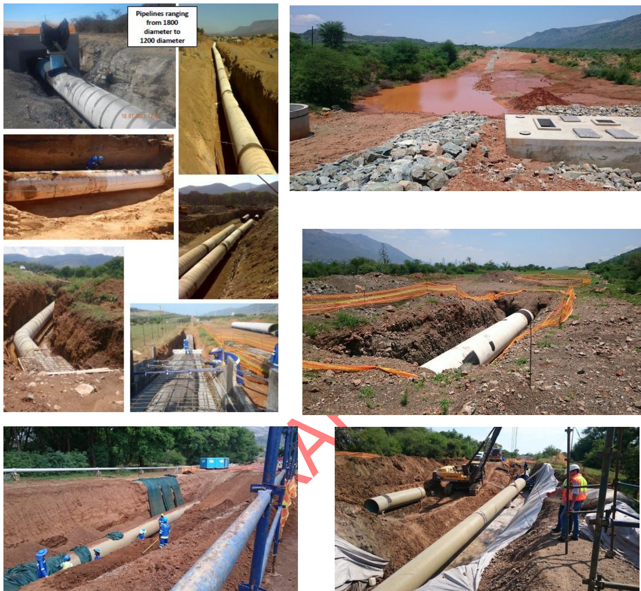
Photo plate 5: Images showing the construction of the bulk water supply pipeline – Phase 2C (Various sources)
