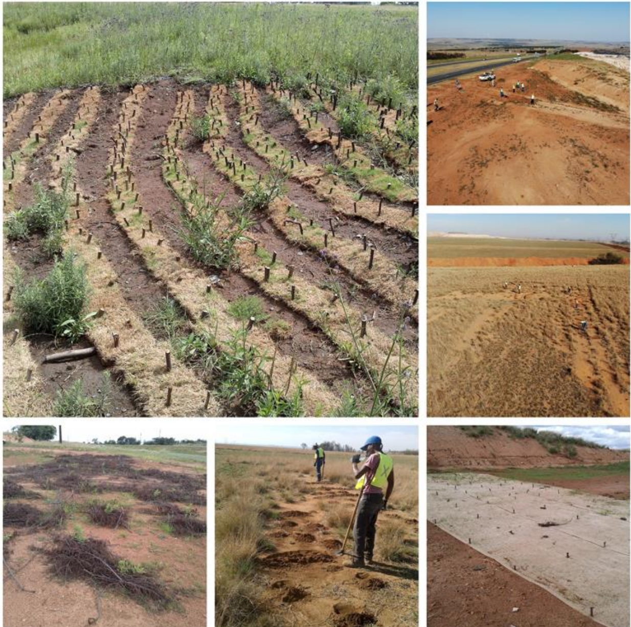
Photo plate 7: Soft manual labour-based techniques used to improve water infiltration and – retention in bare patches (EkolInfo CC Dragline walkway 2019 – 2022)
