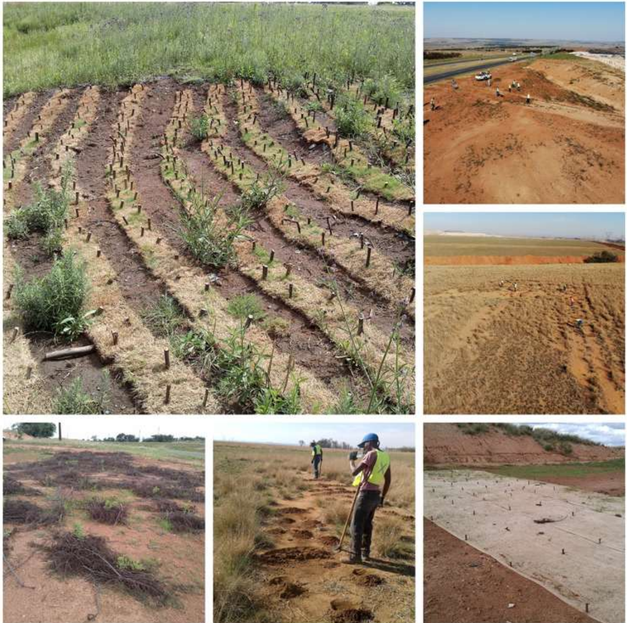
Photo plate 10: Soft manual labour-based techniques used to improve water infiltration and – retention in bare patches (EkolInfo CC Dragline walkway 2019 – 2022)
