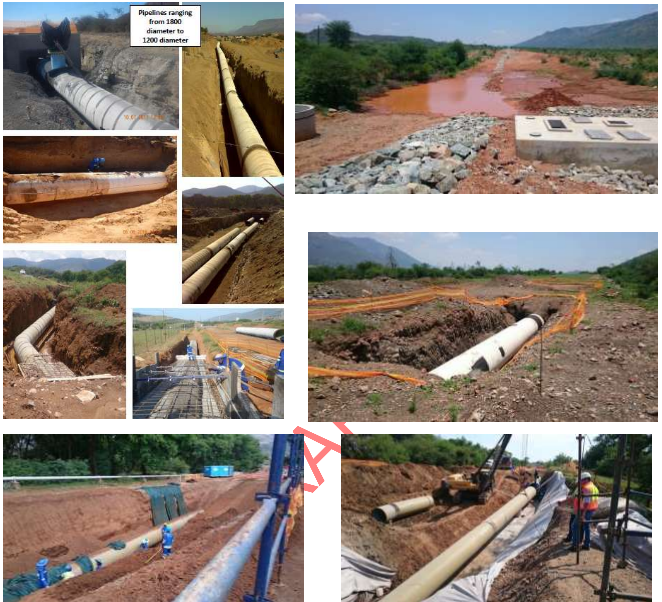
Photo plate 8: Images showing the construction of the bulk water supply pipeline – Phase 2C (Various sources)
