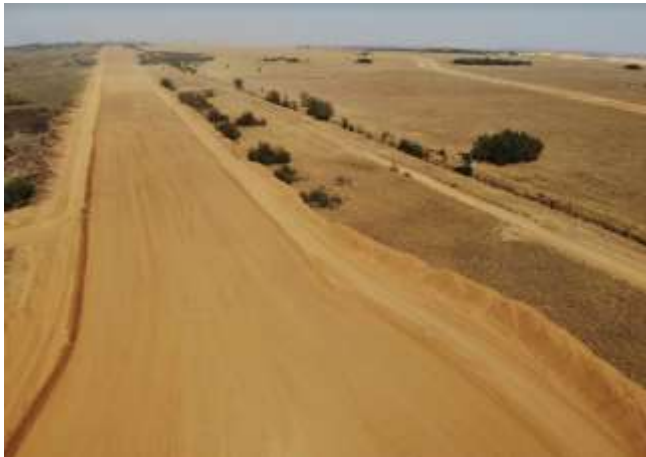
Start of dragline walkway – topsoil separated from subsoil (EkolInfo CC - Aug 2019)
