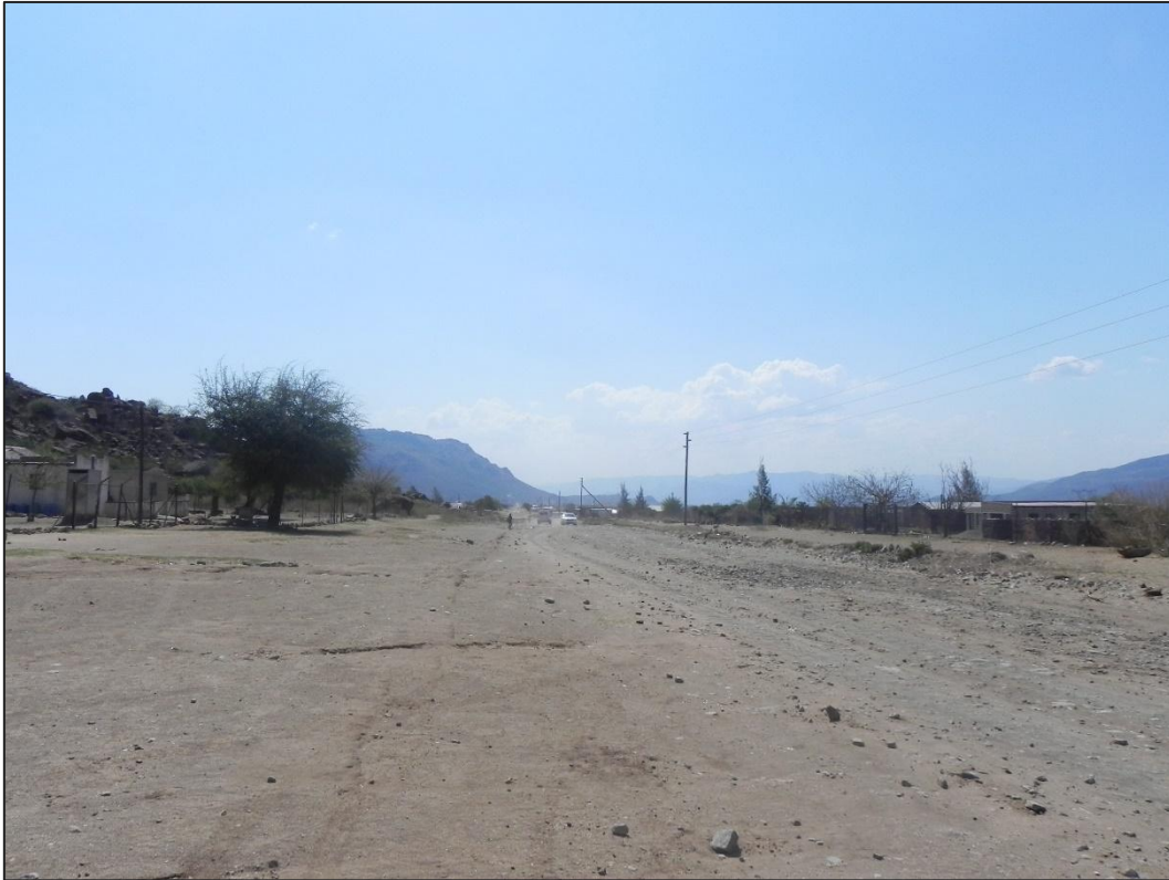
Figure 17: Typical view along the D4180
