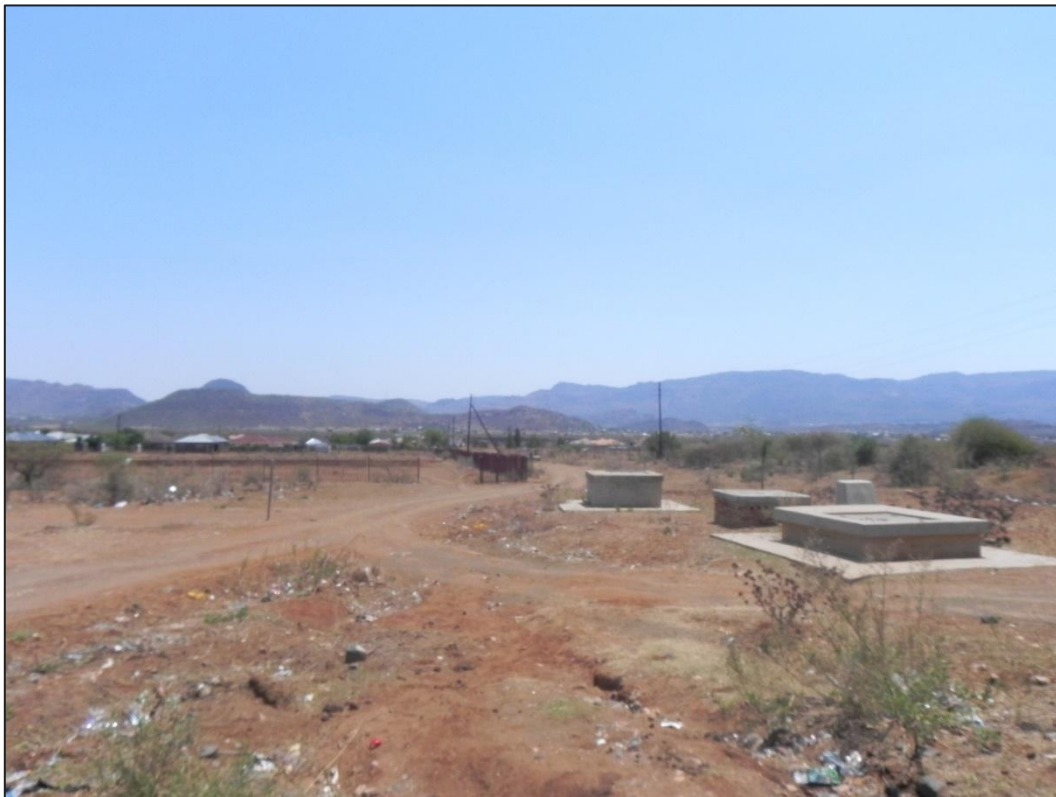
Figure 12: Scour boxes next to the R37, at the eastern section of the alignment
