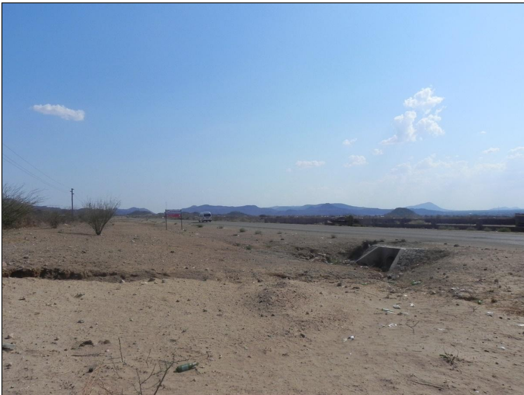
Figure 20: View along the D4190
