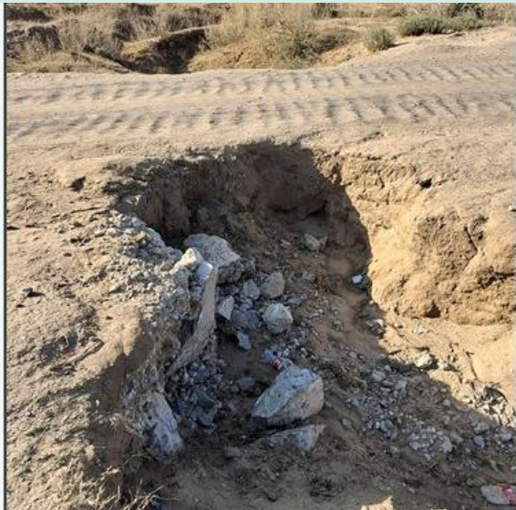
Gravel Road Deterioration at Culvert Crossing
