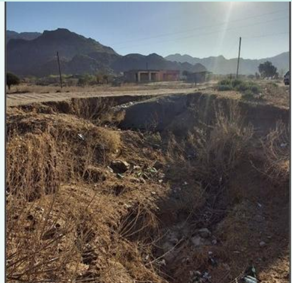
Gravel Road Deterioration at Culvert Crossing
