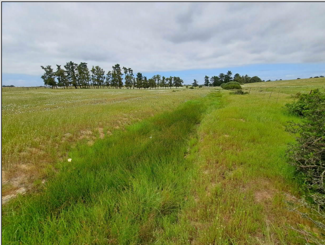
Figure 7 Channelised watercourse as it runs downstream of the R304, towards a farm dam.
