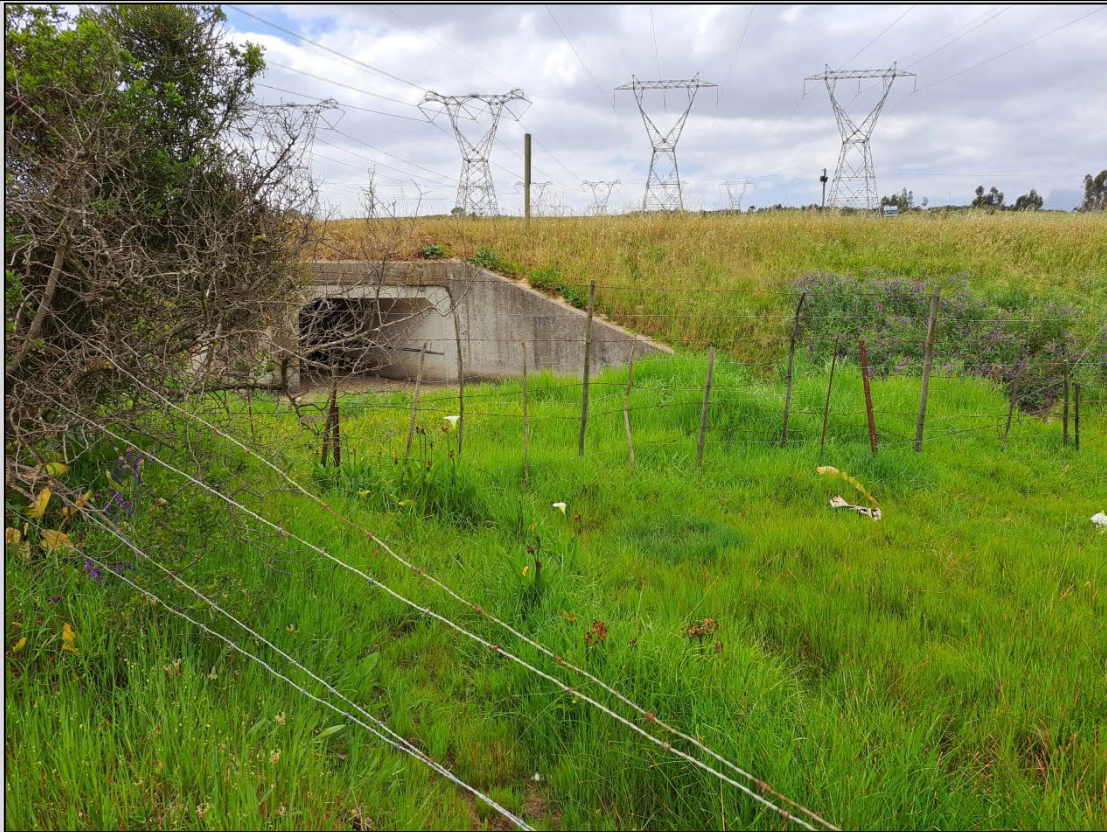
Figure 6 Culvert under the R304, carrying the watercourse (Aquatic Ecosystem 3) under the road.
