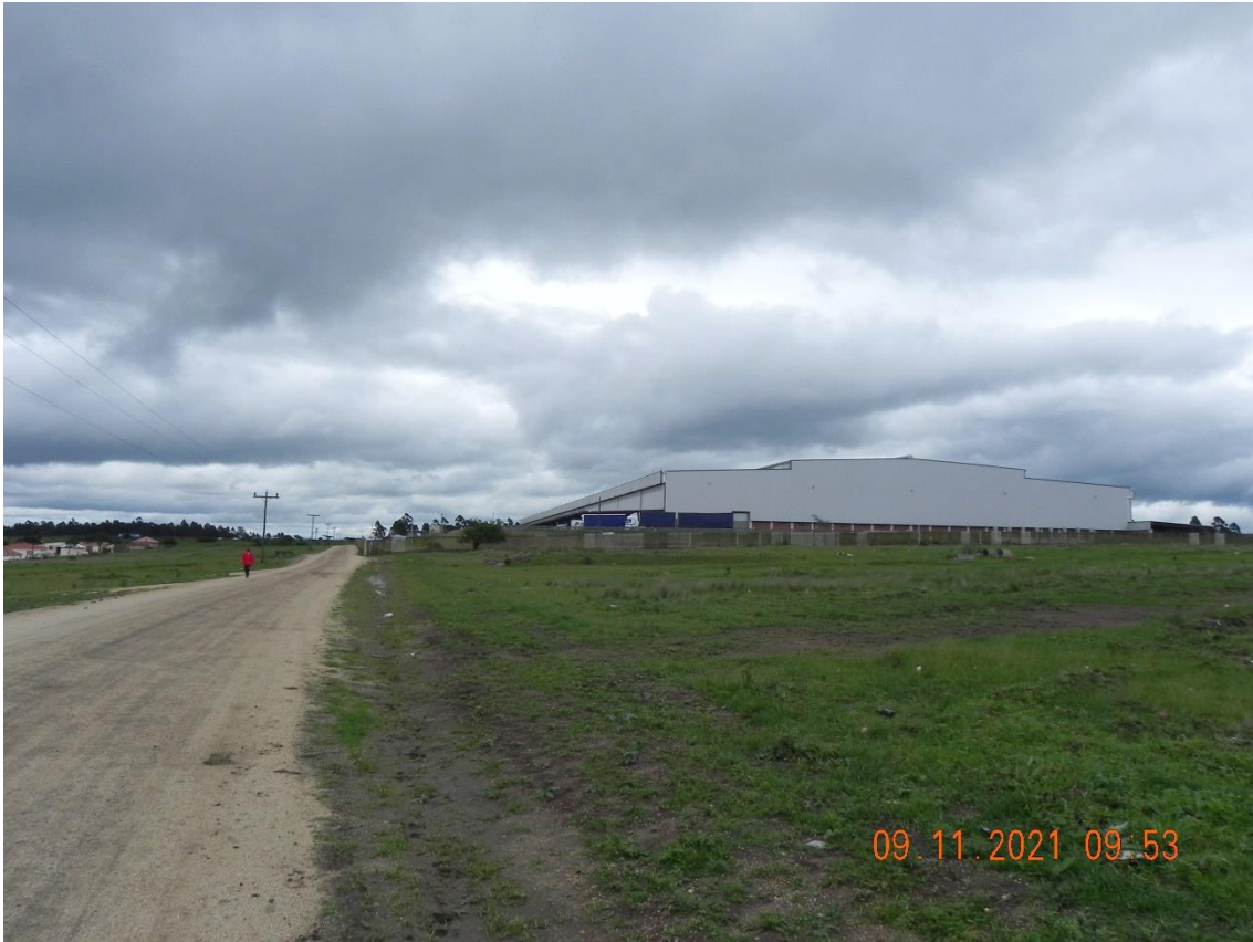
Figure 8: Existing logistic warehouse along the R103 Road
