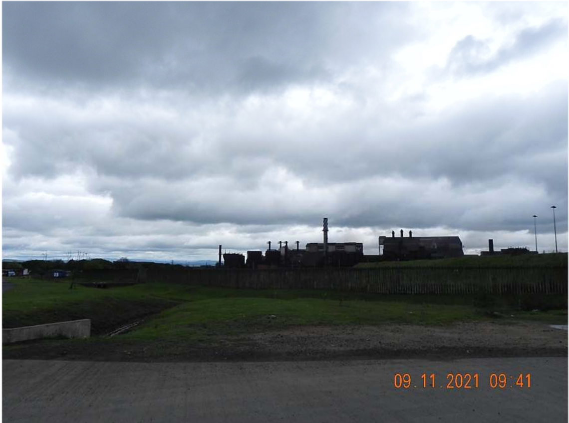
Figure 6: Existing Assmang Cato Ridge Works
