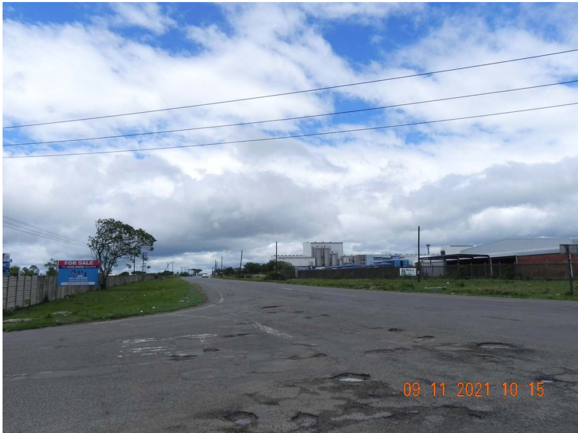
Figure 11: SRF Felxipak (light industrial) along Eddie Hagen Drive
