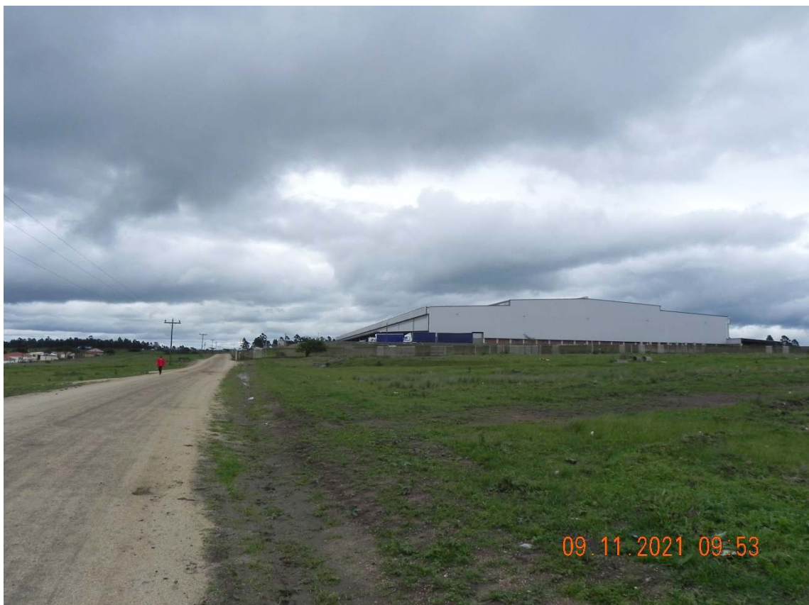
Figure 8: Existing logistic warehouse along the R103 Road
