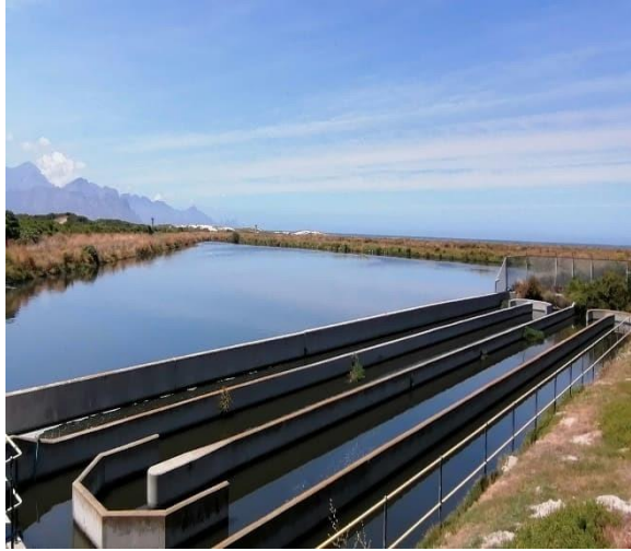
Chlorine Contact Tank
