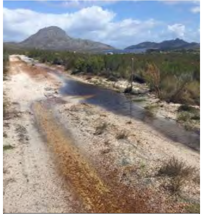
Figure 3.9 Example of diverted runoff caused by the roads that bisect wetlands and result in drying out of wetlands downslope of the road.
