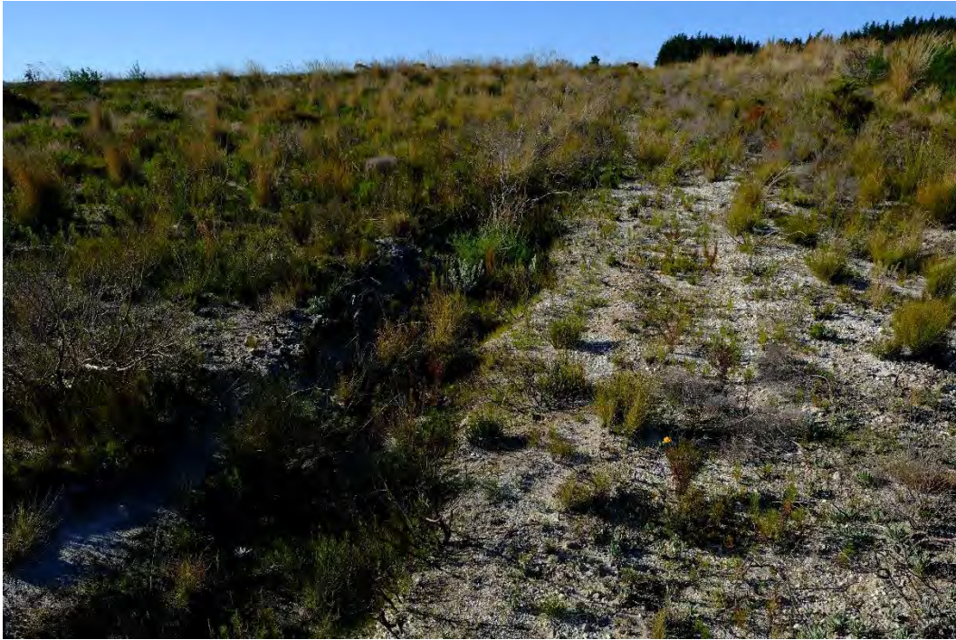
Plate 2: View of H1A5, looking east. The whitish area on the centre and righthand side of the picture is the old road surface, now partly rehabilitating.
