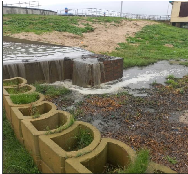
Splitter boxes overflowing
