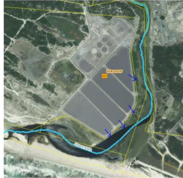
Figure 1 Maturation pond embankment scour protection, and groundwater seepage toward the Eerste River to be addressed in the SMP.
