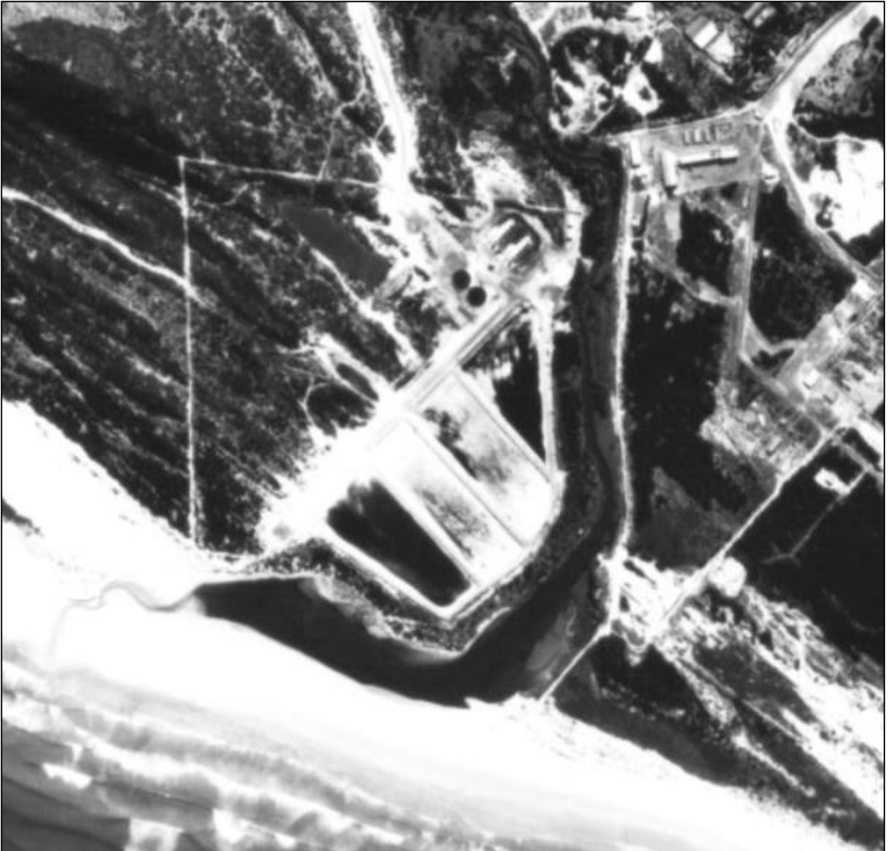
Figure 21: 1978 aerial photograph showing the first wastewater treatment works in place.
