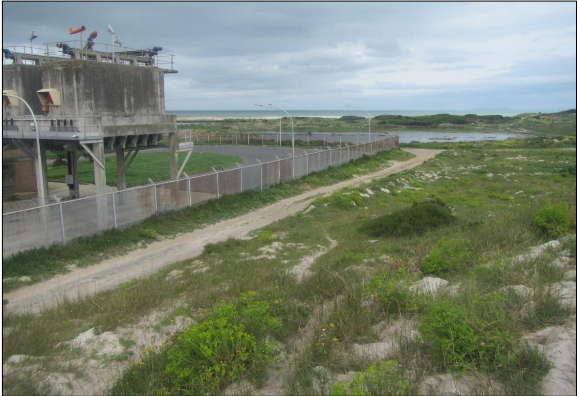
Figure 11: Looking south across the western corner of the existing WWTW.
