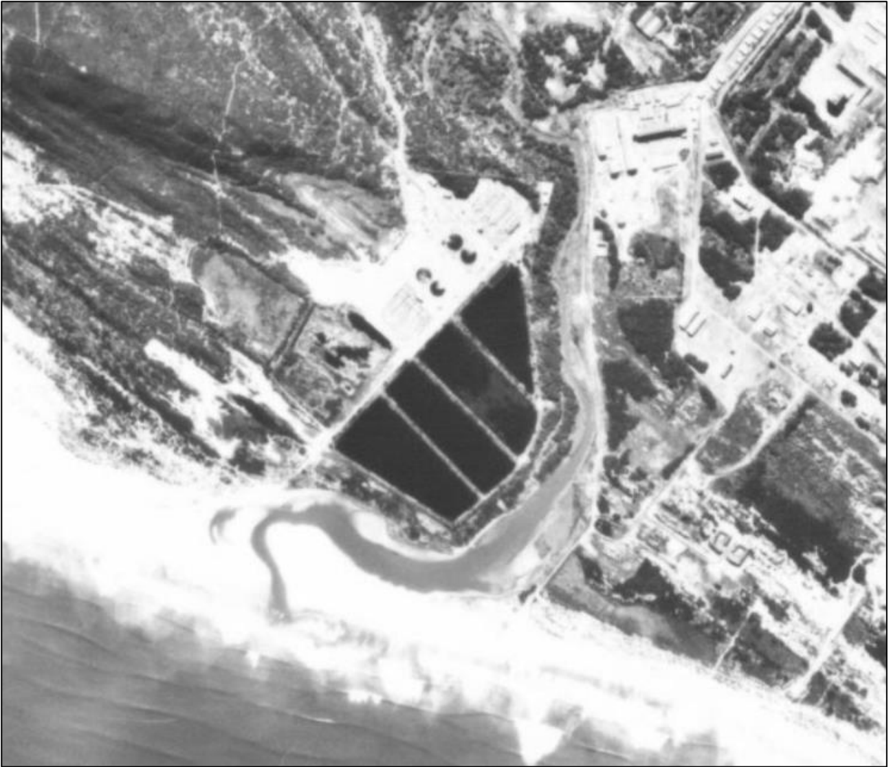
Figure 22: 1989 aerial photograph showing the wastewater treatment works to have been expanded to its current size.
