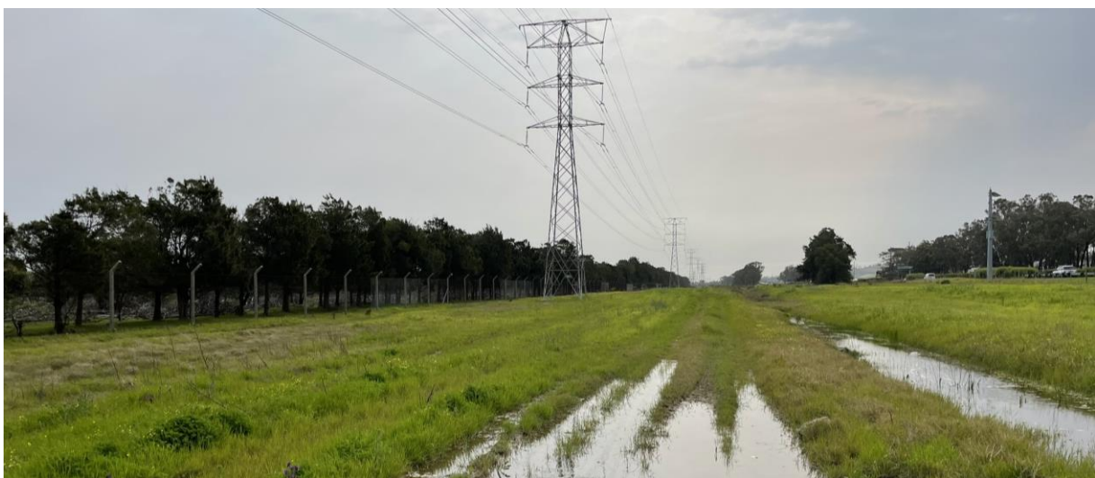
Figure 12. View of the floodplain wetland at the N2 Highway within the existing Eskom powerline corridor.
