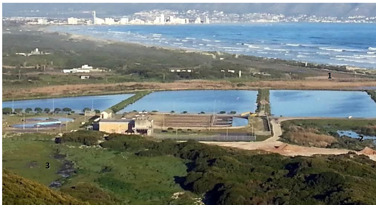
Figure 20. Aerial photograph of the wetland areas adjacent to the Macassar WWTW
