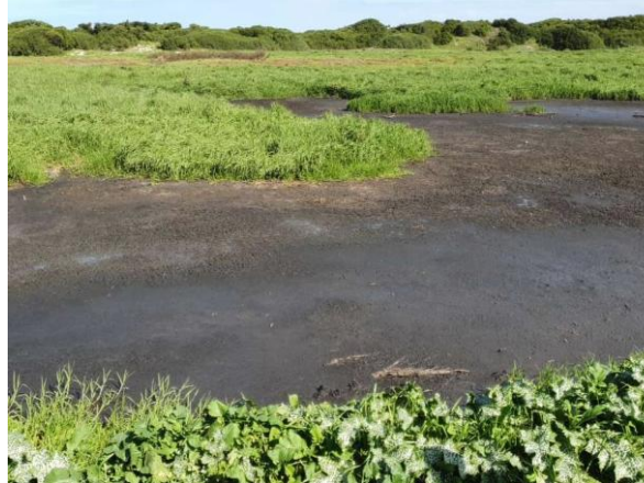
Old Sludge Lagoon
