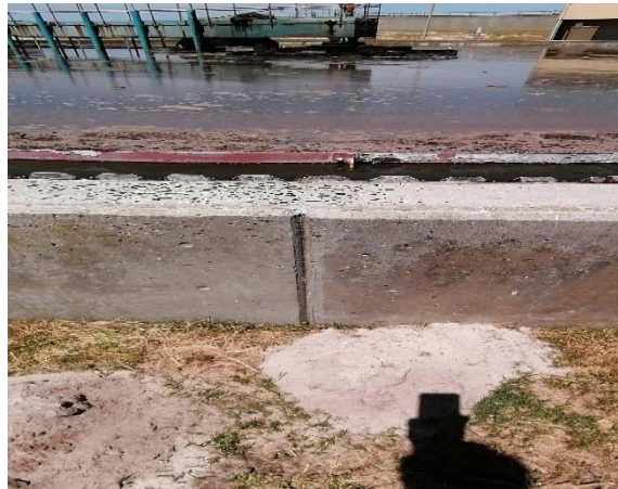
Secondary Settling Tank
