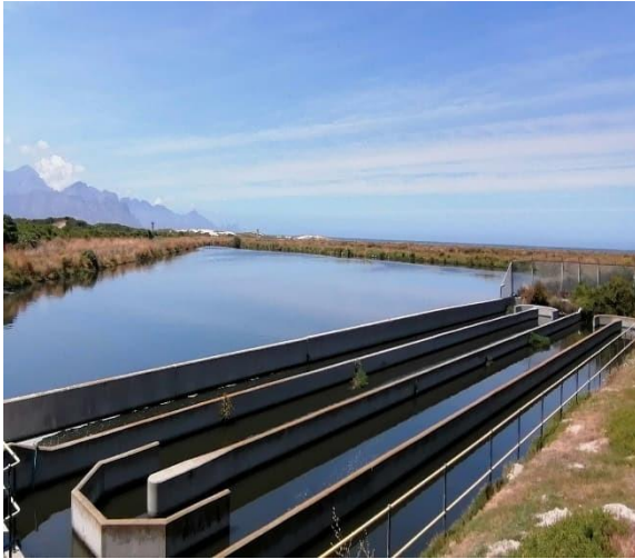
Chlorine Contact Tank
