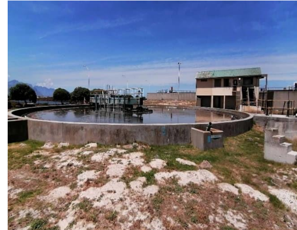
Secondary Settling Tank
