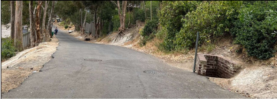
FIGURE 4: HUGHENDEN ROAD ABOVE ERF 2596 SHOWING STORMWATER INFRASTRUCTURE WHICH INTERCEPTS RUNOFF FROM ABOVE THE SITE
