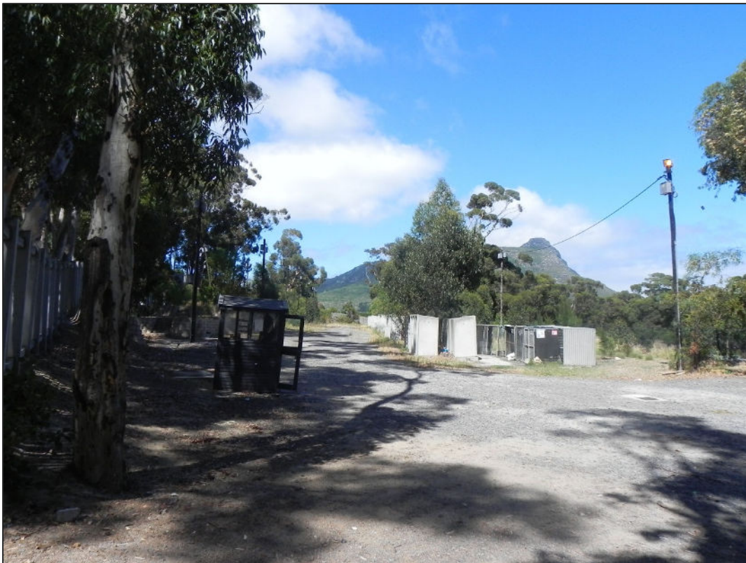
Figure 10: Existing concrete structures and temporary security house on site
