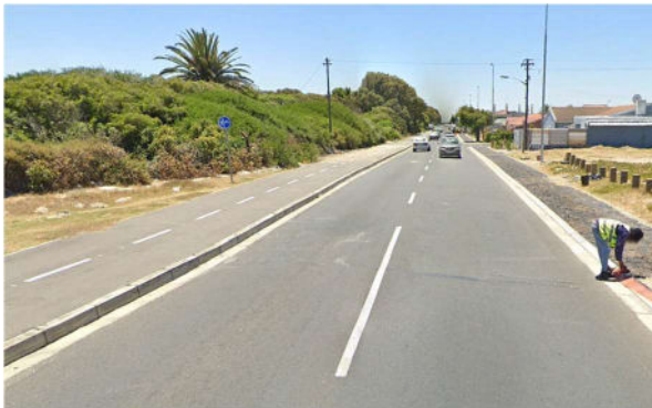
Figure 11: Existing NMT facilities along Klip Road, northbound
