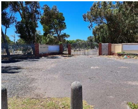
Figure 20: Closed access gate to cemetery from De Waal Road, Access 1
