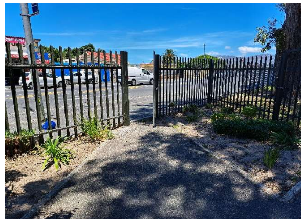
Figure 21: Pedestrian gate from Klip Road, Access 4
