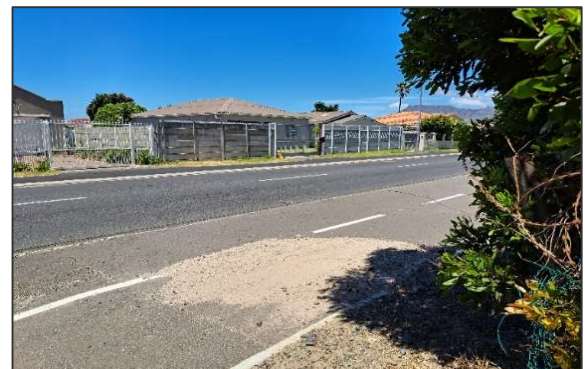
Figure 12: NMT Facilities along cemetery along Klip Road, southbound
