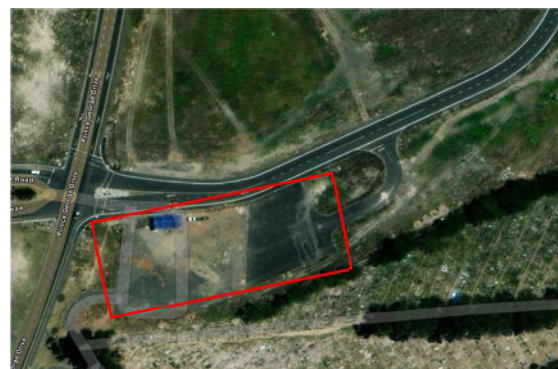
Figure 15: Existing gravel parking along De Waal Road
