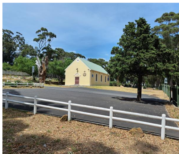
Figure 13: Existing Parking lot
