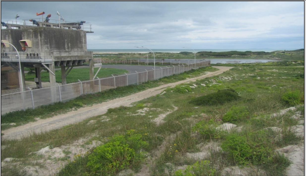
Figure 14: Looking south across the western corner of the existing WWTW
