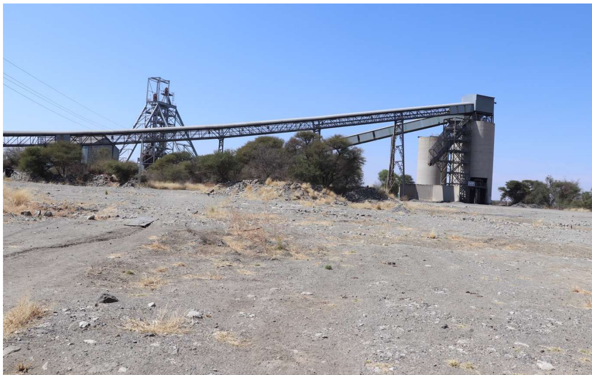
Figure 8-13: This conveyor and concrete silos are located immediately outside the study area but provide an indication of the mining-related activities which had taken place in this area.
