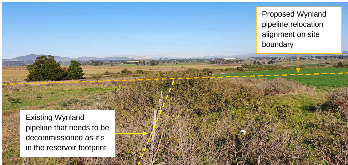
Figure 22 View of the middle of the reservoir site where the Wynland pipeline will need to be relocated, looking south west
