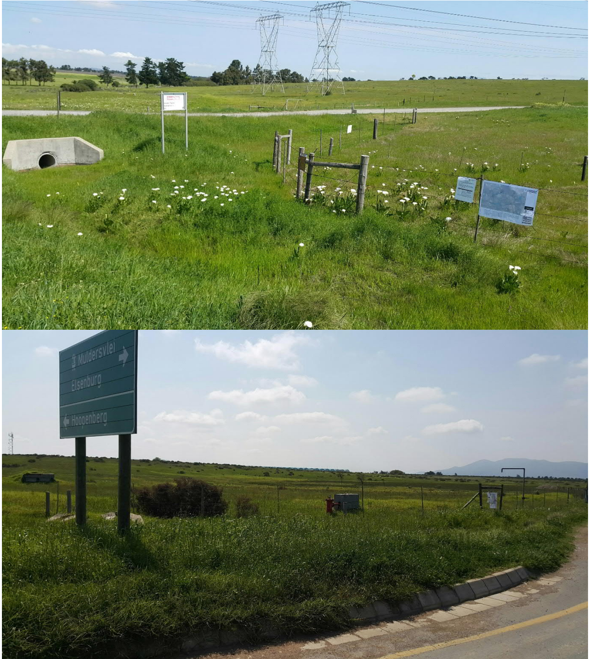
Figure 1 - WULA notice on property RE/1370 (County Fair) - intersection with R304
