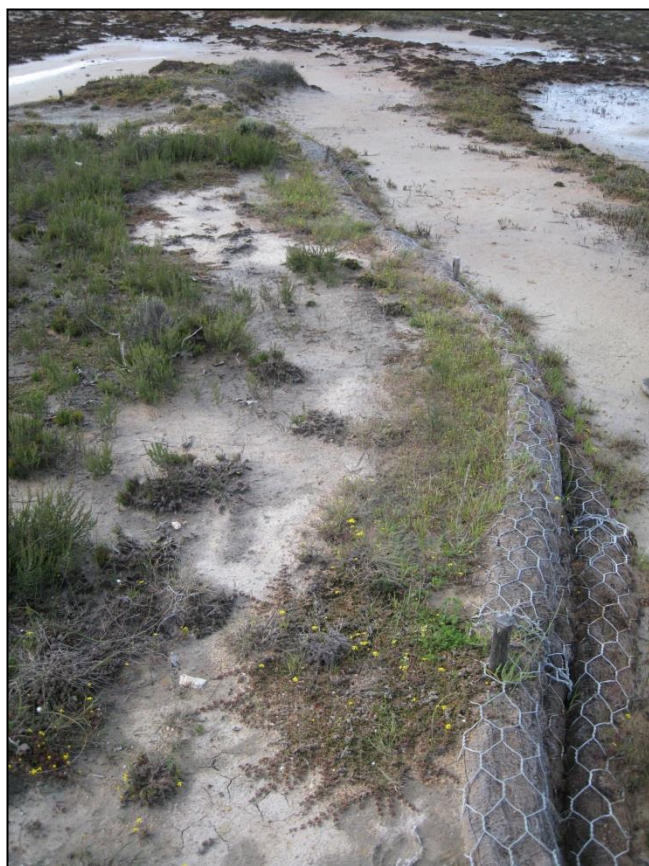
Figure A4.8.13 Ecologs installed for stabilisation.
