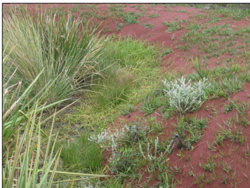
Figure A4.8.14 Banks stabilised by geofabric, showing natural re-growth of indigenous species through the mat.
