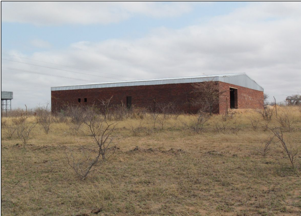
Figure 36 – Closer view of the contemporary brick structure.
