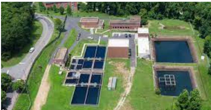
Figure 4: Typical example of a bulk water treatment works.
