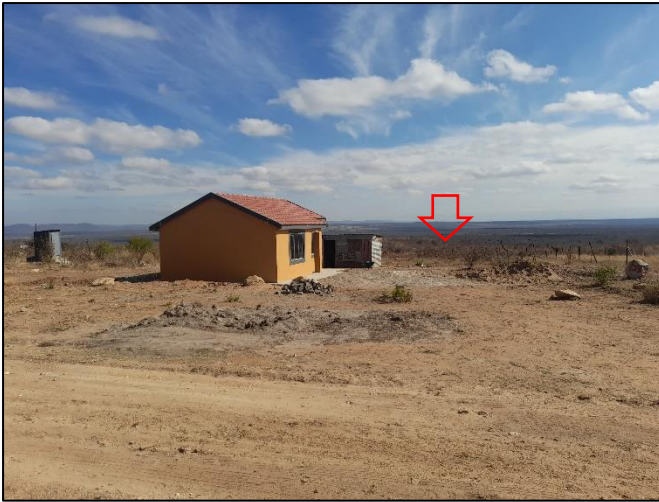
Figure 7: View from the Sekuruwe settlement directly south of the proposed Sekuruwe WTW. Due to the Sekuruwe WTW situated directly adjacent to the settlement, the residents in this portion of the settlement will have direct views of the proposed infrastructure (red arrow).
