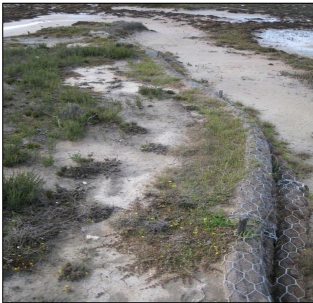
Figure 5.2 (Left) Ecologs used to stabilise the banks of a stream; (Below) Geotextile stabilisation of a slope.
