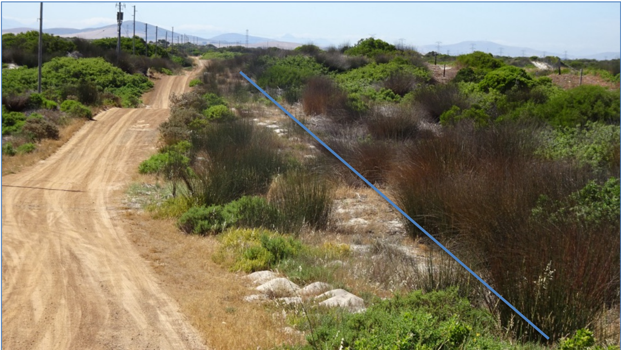
Figure 13. Pipeline disturbance footprint visible (blue line) in the Witsands Aquifer Nature close to the R27 showing degraded CFDS. The blue line represents the pipeline.
