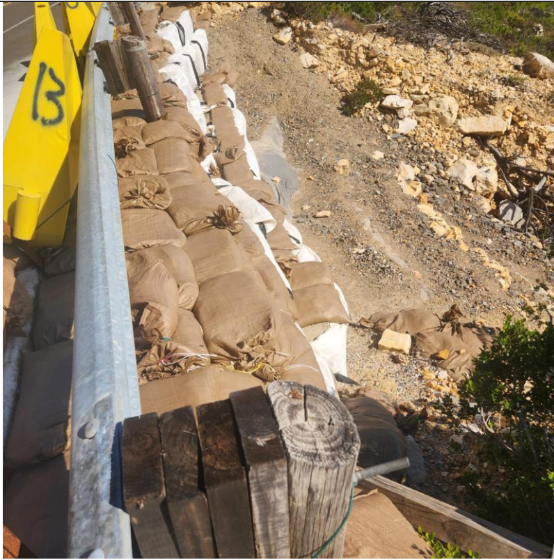
Temporary roadside reinforcement using sandbags and barriers to prevent further erosion of slope 1 along the Steenbras WTP access road
