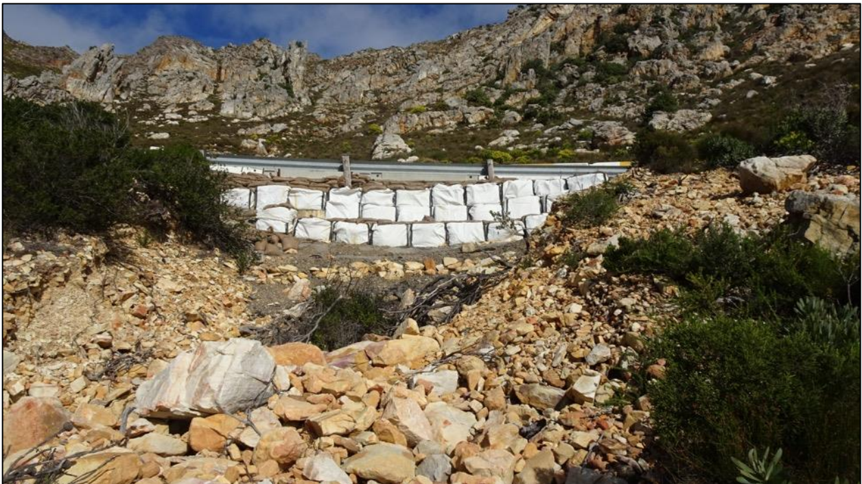
Figure 19. Sand bags used to temporary repair the built the eroded road edge.
