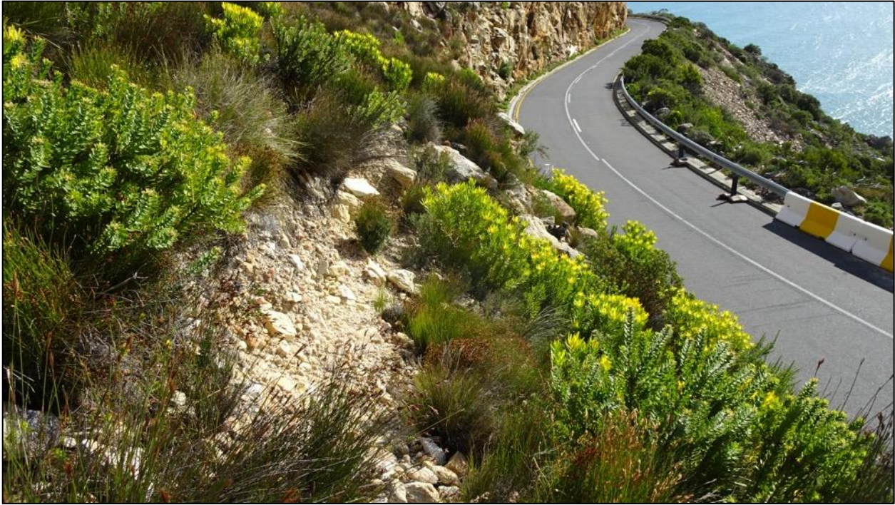
Figure 15. Some erosion with very loose substrate just upslope from the road at waypoint 010 (34°10'38.46"S; 18°50'18.26"E).
