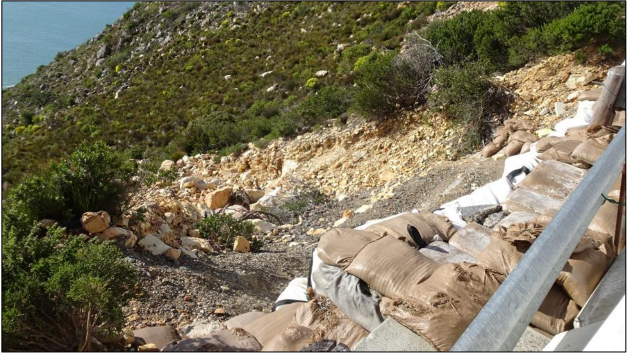
Figure 18. Looking downslope from the road edge.
