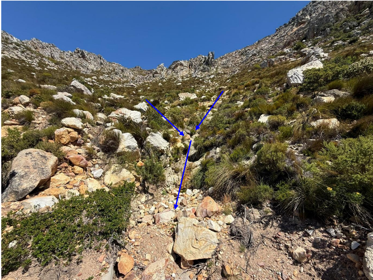
Figure 3. View of the watercourse at Slope 1, upslope of the Steenbras WTP access road.
