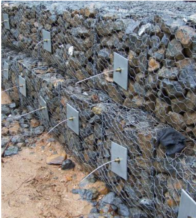
Figure 12. Example of an anchored gabion wall
