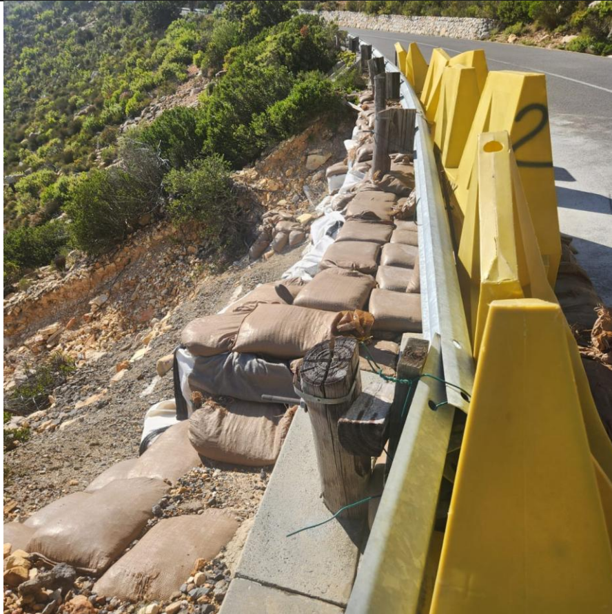
Temporary roadside reinforcement using sandbags and barriers to prevent erosion and support slope stability on the proposed rehabilitation area
