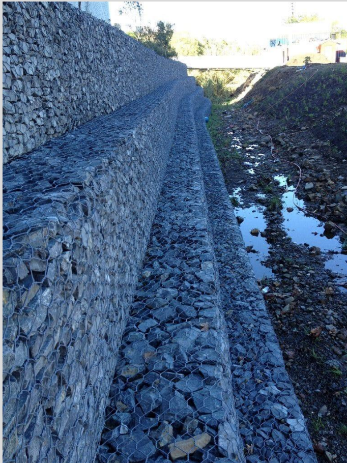
Figure 16: Example of gabion structures. Source: (Gabion Baskets, 2026)
