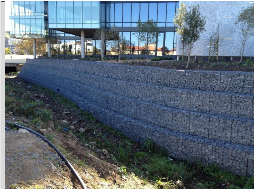
Figure 17: Example of gabion structures. Source: (Gabion Baskets, 2026)
